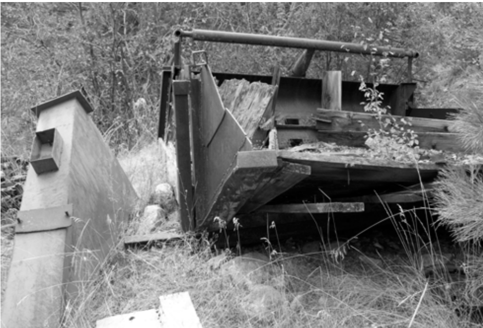
The huge sluice above has a metal and wood bottom with the necessary riffles. The pipe across the top has holes to spray water down on the gravel as it was travelling through, ensuring all of the black sand and gold would be washed into the riffles.
