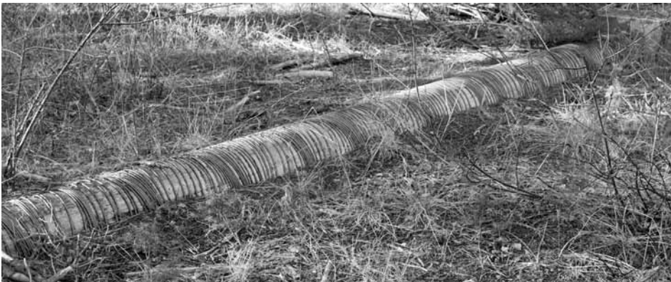
Gord Davis gave directions to find this still useable, but abandoned, irrigation system. A couple of hundred feet of wooden pipe were fed by a now dry irrigation ditch and once supplied water to a local ranch. Photo courtesy Richard Forrest
