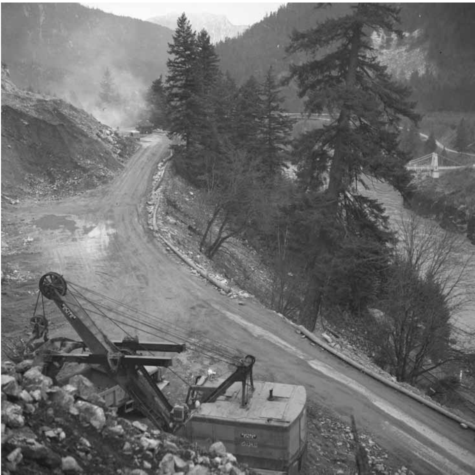
Above: A Bucyrus Erie Model 54-B diesel shovel clears the new right-of-way. A large machine for the time, it could handle 2½ cubic yards per bucket load. A large dump truck is just visible rounding the corner at the far end of the new road. The old Alexandra bridge is visible to the right, while the new Alexandra bridge is just visible between the trees above it. The condition of the roadway leading into Spuzzum at the far end of the suspension bridge suggests that traffic is still using the old road.
