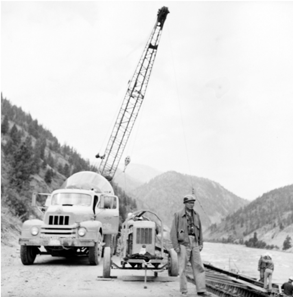
Above: A concrete truck is off-loading to a crane to place concrete into the formed wall at the right. It is possible that this photograph records the construction of the retaining wall at the s-curves below Tank Creek Hill on the Thompson River.
