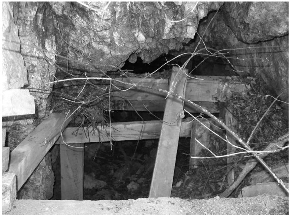
The Rosyd Mine in 2005 — more overgrown and more fallen rock.
