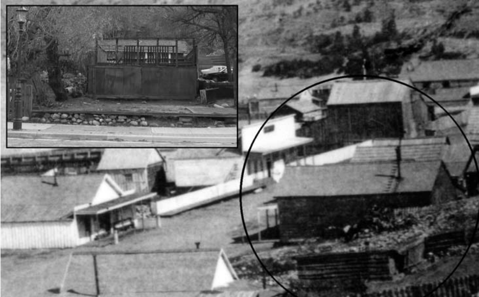
Rebagliati freight shed (circled) in 1890, and being torn down in 2006 (inset).
