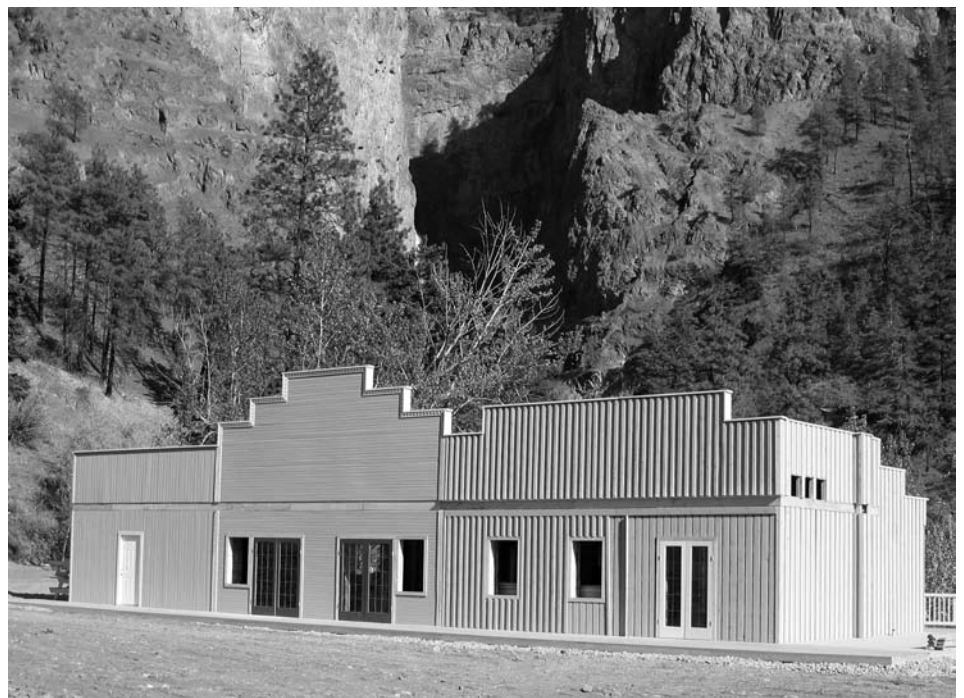
Kumsheen's Nicomen House under construction in early 2006.
