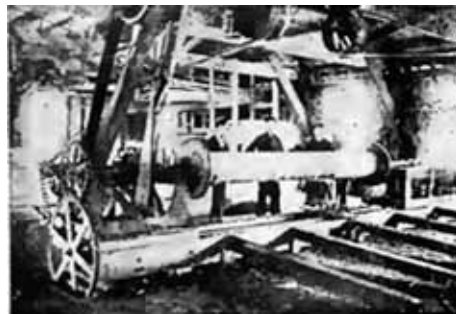
Pipes being wound with wire at the Dominion Wood Pipe Co. - 1908
